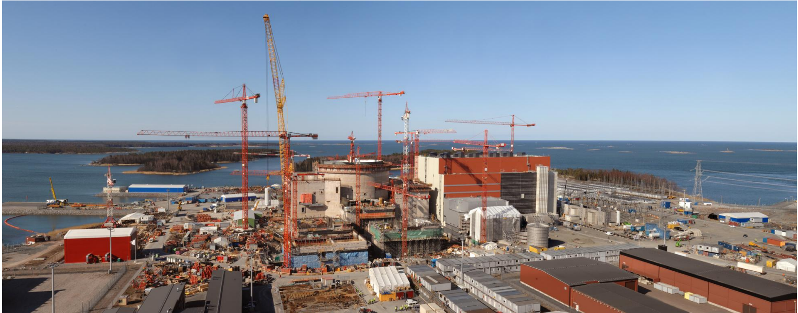
Olkiluoto 3 in April 2009
